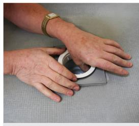
Screw the white plastic ring through the Showerlay into the Dallmer drain below. To do this, reach your thumb through the hole and lift the drain up to the thread.
