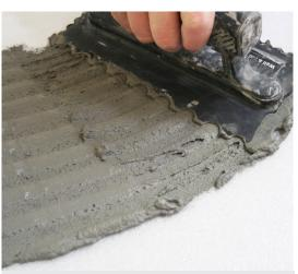
Now fix down the Showerlay to the Plinth once again using a full bed of flexible cement based tile adhesive.
