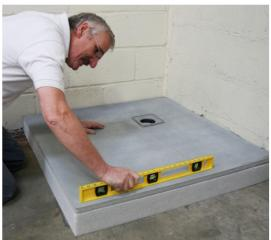
It is critical to make sure the Showerlay is level on all edges to ensure that when being used, all water will drain away.
