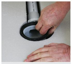
Connect the Dallmer drain to the pipe, feed through the wall. Allow the drain enough space to move freely up and down. Check that the black rubber ring is on top of the drain.
