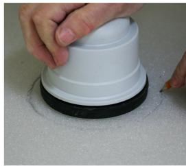
4 Remove the Showerlay and place the Dallmer drain upside down over the circle drawn on the Plinth. Now draw a pencil line around the Dallmer drain leaving roughly a 10mm gap.
