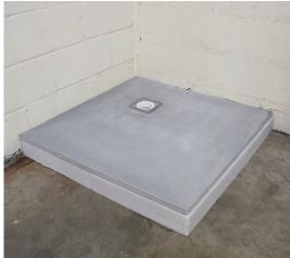
**16** You can also apply Marmox Multiboards to the surrounding walls and floor. Now it is ready to tile and to add the desired show enclosure.
