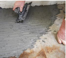
**8** Now fix down the Plinth to the floor using a full bed of flexible cement based tile adhesive. Use the adhesive to help level any uneven floors.
