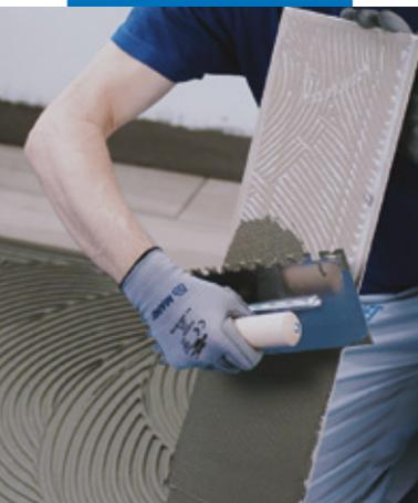
Install ceramic or stone tiles with a suitable MAPEI adhesive of at least C2 class
