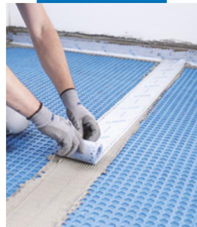
*Waterproofing of joints between the sheets with Mapeband Easy, bonded with Mapeguard WP Adhesive*
