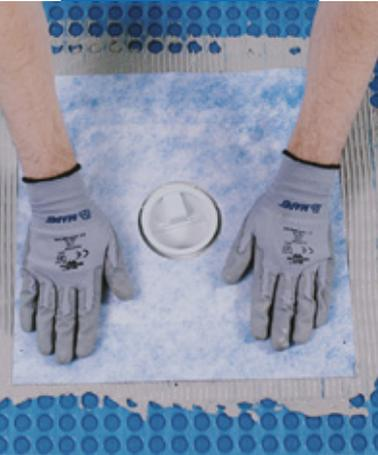
Waterproof drains with Drain Vertical/Drain Lateral
