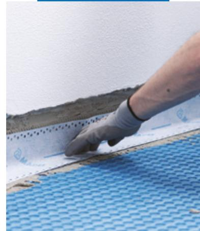
*Perimetral waterproofing with Mapeband Easy, bonded with Mapeguard WP Adhesive*
