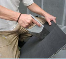
**2** It's easy to cut the SoundBoards with a knife or saw. Cut the first board of every other row in half to allow the joints to be staggered.
