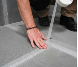
Then apply 'Marmox Reinforcing Tape' over all the joints. For wet areas use 'Marmox S/A Waterproof Tape'. Now the floor is ready to be tiled.
