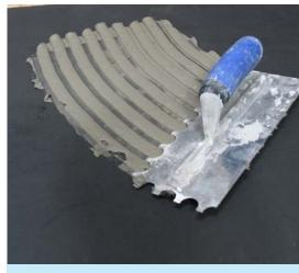
4 Alternatively you can comb on a full bed of cement based flexible tile adhesive.
