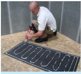
**3** Apply Marmox Multibond to the black rubber side of the Sound Board.
