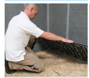
**5** Leave a gap of 5mm around the edge of the room where the floor meets the walls. Lay the SoundBoard rubber side down onto the floor and press down firmly.
