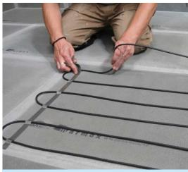
**8** If using undertile heating, apply the heat wire directly to the SoundBoard and then tile over the top.
