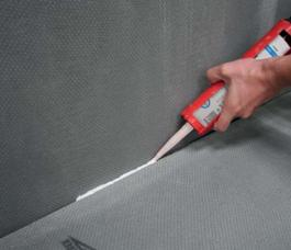
6 It's important to squeeze some Marmox Multibond in the 5mm gap around the floor at the base of the walls.
