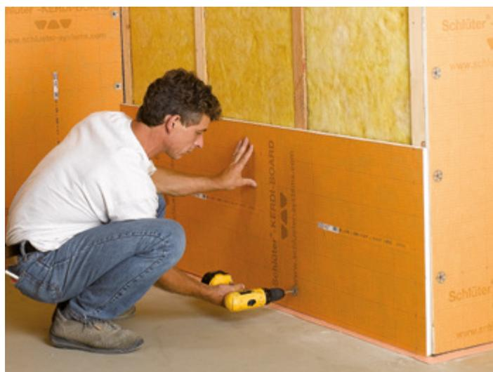
Stud frame structures made of wood or metal are typically covered with drywall or wooden panels. However, such materials are typically unsuitable as tile substrates, particularly in areas of high moisture.
